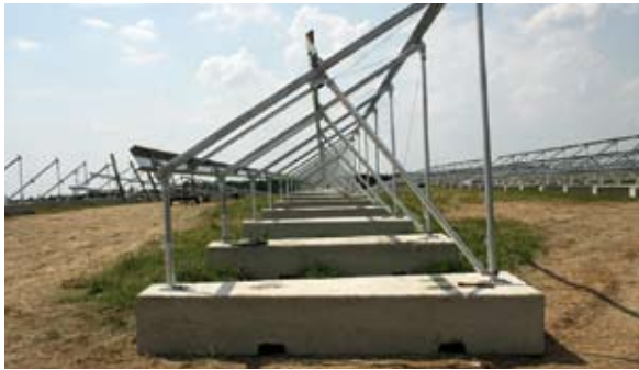
Concrete block foundation: individually designed foundation technology especially for waste dumps which ensure, that the foil will not be damaged.
