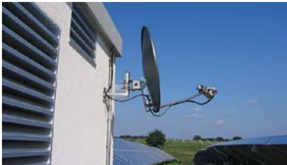
The solar park is monitored using remote data transmission methods and monitoring software which offers a high level of internet support.
