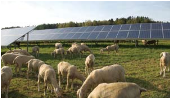
The vegetation in the solar park Pfeffenhausen is controlled by grazing sheep. This keeps the area in agricultural use.
