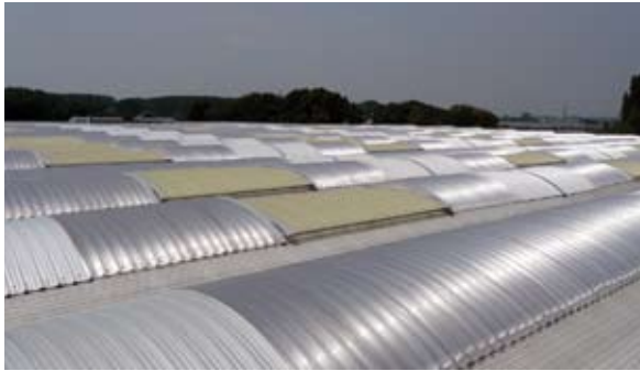
This PV roof top is a case sui generis. The mounting system is an in-house development of Scatec Solar's engineers.
