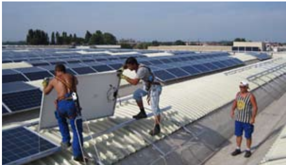
Before the Milano project, it wasn't possible to install PV modules on roof tops with barrel vault roofs. This unique customized solution could be realized for the first time.
