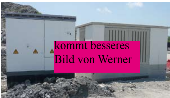
Electrical design in the solar park: 25,938 solar modules laid out in 1,179 strings. 9 outdoor inverter stations and MV-transformers. Each has a transformer station.
